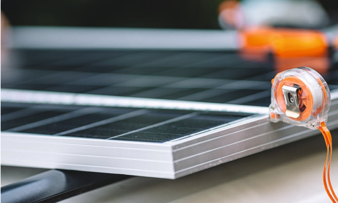
Necessary precision work, the construction of PV systems. Photo: Newpowa, Unsplash
